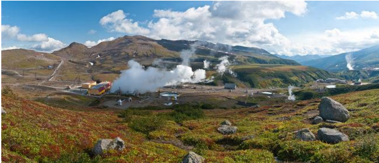
Figure 10. Mutnovsky geothermal power plant. Photo taken from: http://greenevolution.ru/
